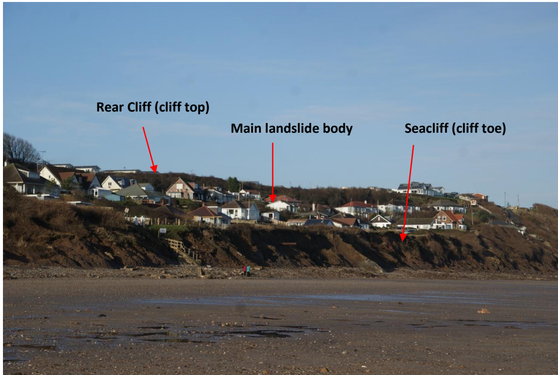
Photo 1 Flat Cliffs: the main landslide complex components
