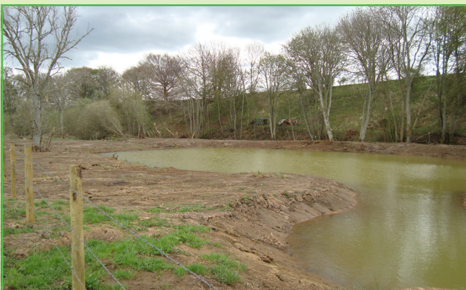
Fig 2 Pond just after completion
