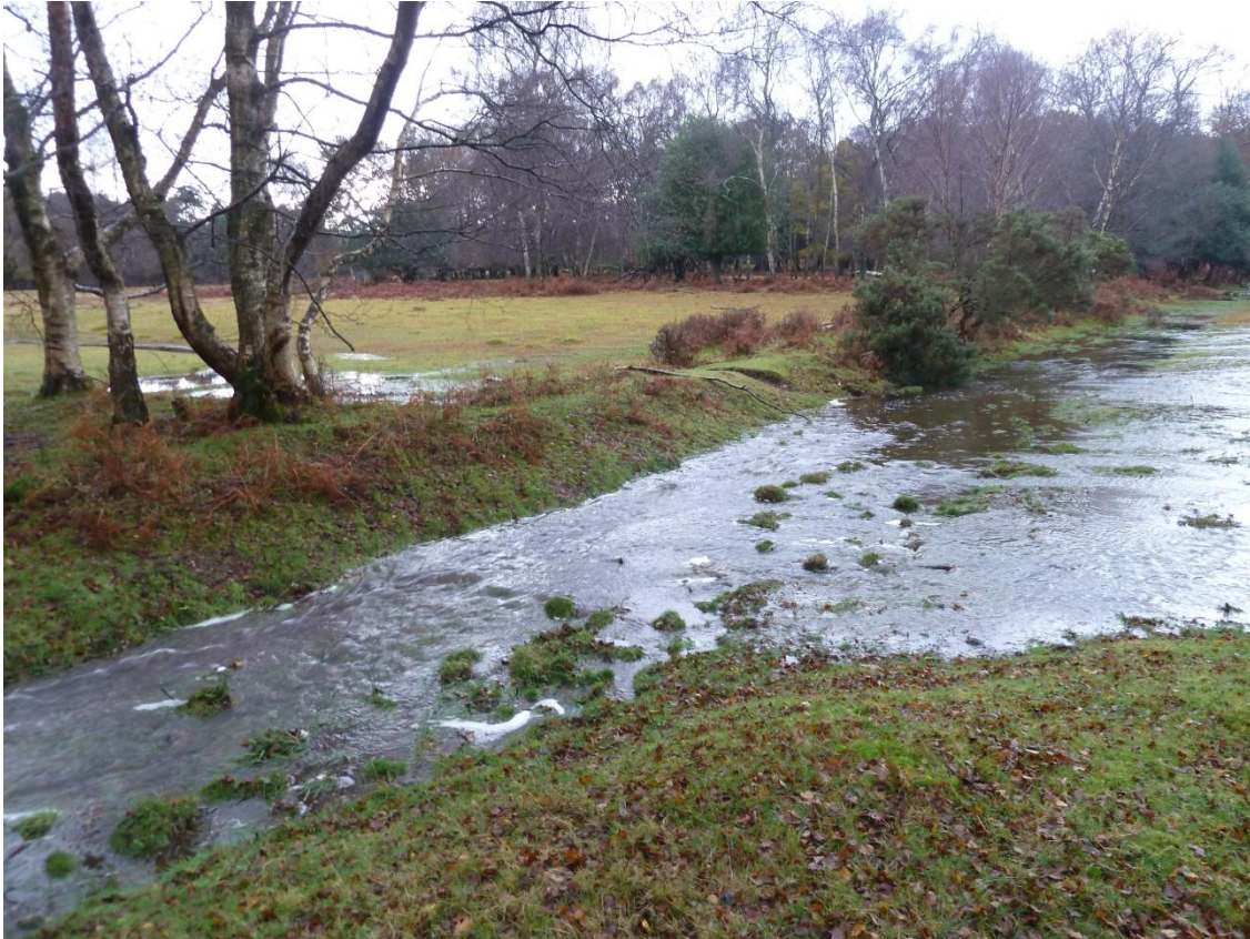
Figure 1-5: Right bank embankment providing obstacle to natural overland flow route
