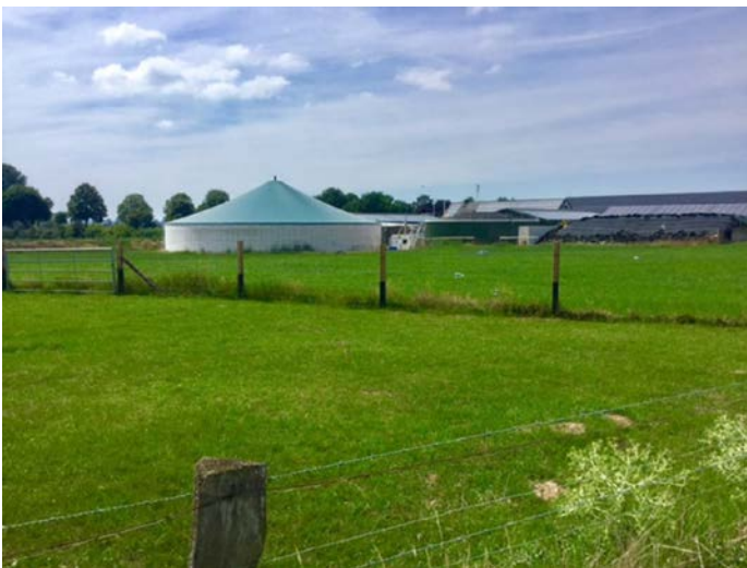
A slurry store cover helps to reduce the loss of ammonia from storage and needs to be part of an overall farm package that considers inputs, usage, storage and recycling to land.
