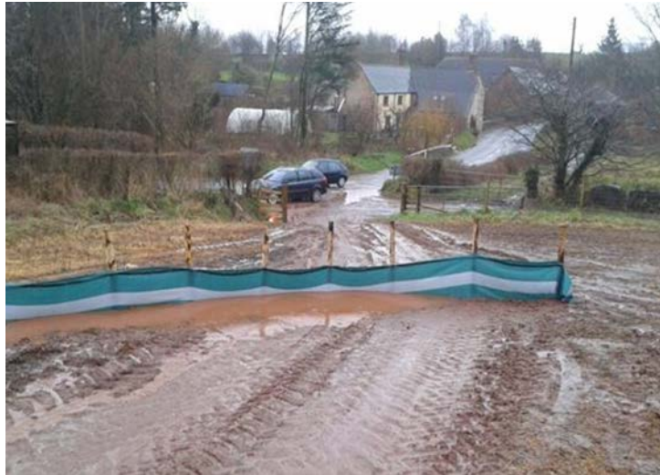
Filter fence helps manage silt and runoff to local roads
