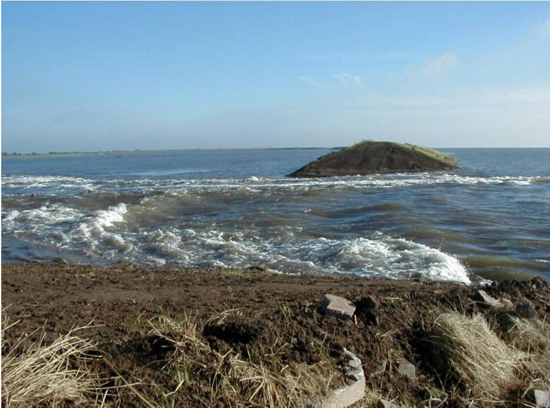
**Figure C.7. Breach at flood tide.**
