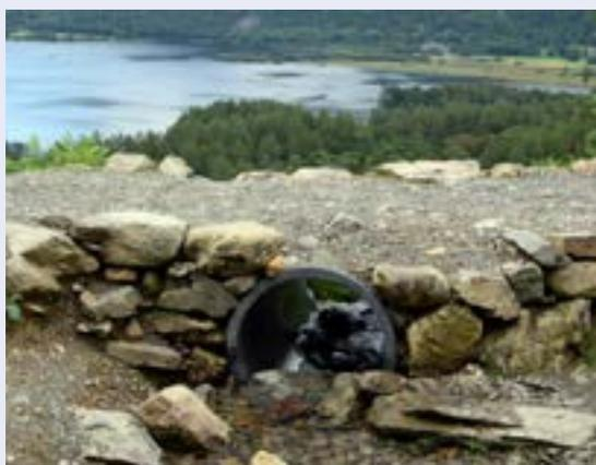
**Repaired section of Cat Bells path with improved drainage culvert.** © Natural England/A Mackintosh
