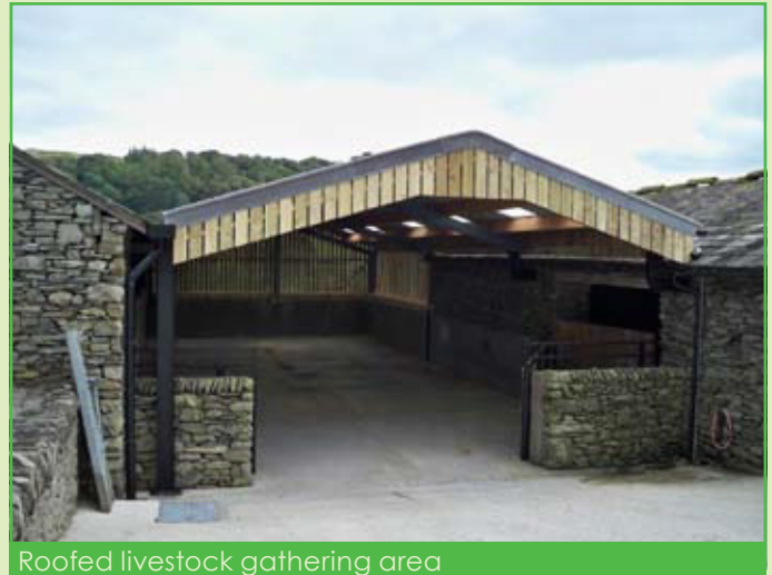
Roofed livestock gathering area
