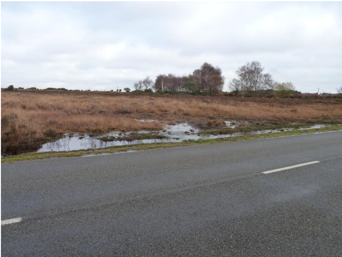
Figure 1-13: Ponding upstream of the road
