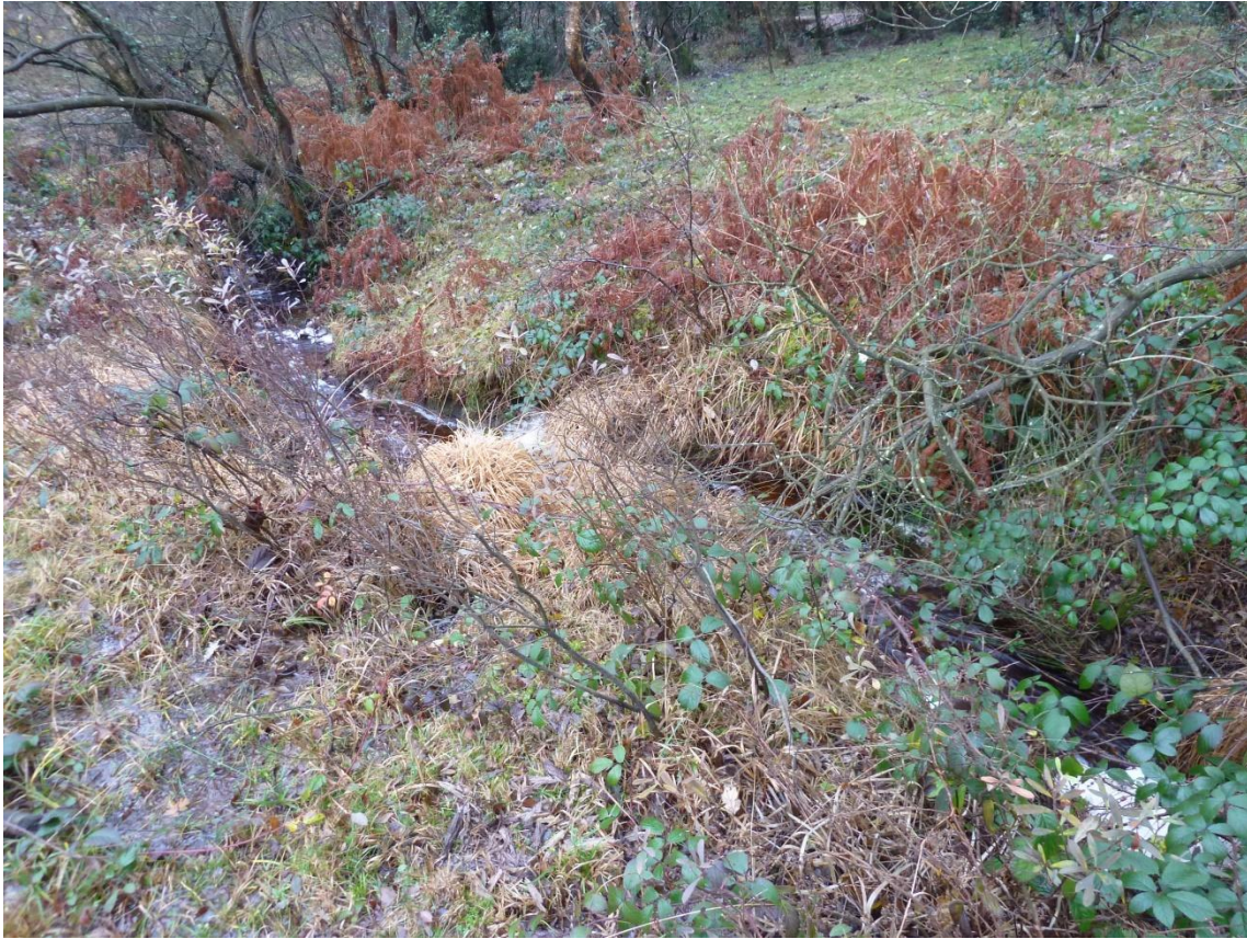
The source of the unit is Beaulieu Heath. Figure 1-5 summarises the existing hydromorphology and pressure impacting unit 422.
