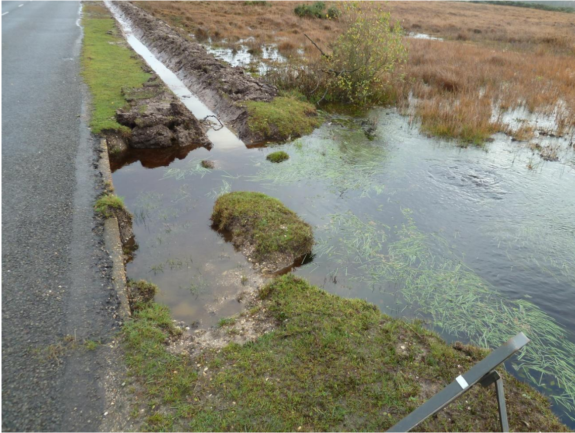
Figure 1-13: Ponding upstream of the road
