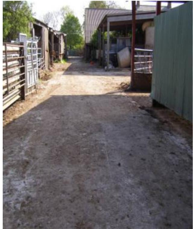
The yard after work completed – new rainwater goods, underground drainage and concreting – making it easier to keep clear of mud and muck.
