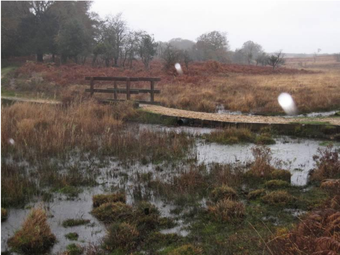
Figure 4-14: Trackway causing localised ponding of water on Soldiers Bog
