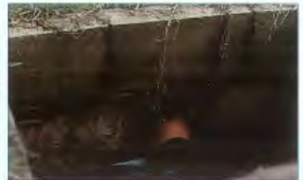
Soil pipe sluice
