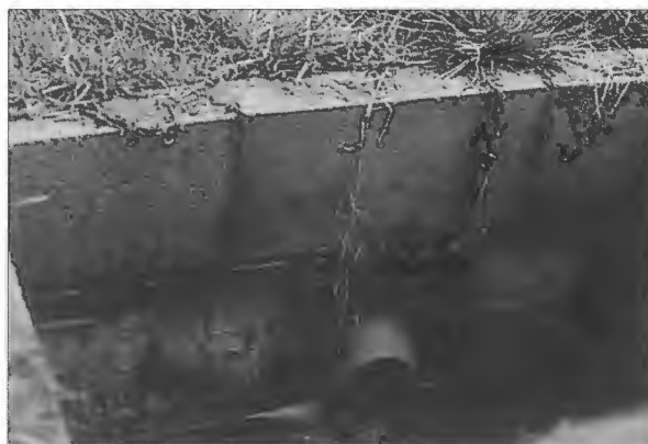
Soil pipe sluice
