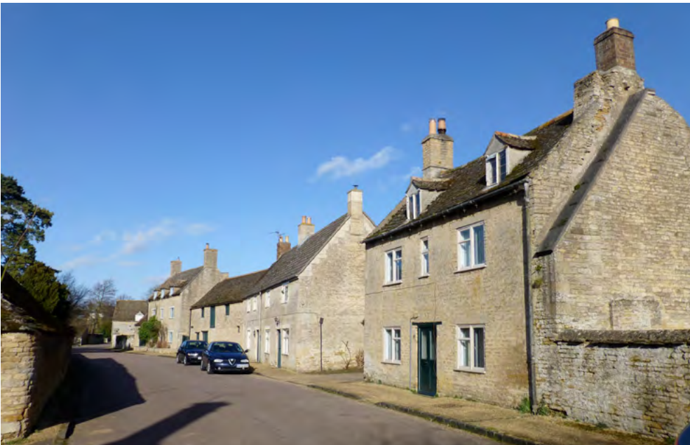
Duddington village high street, typical of the area, with houses built with local limestone and using the heavy Collyweston roofing slates.
