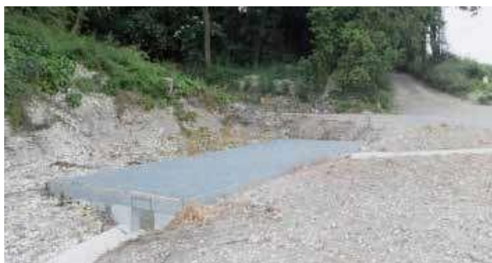
The sediment trap installed in 2012 at the base of the track
