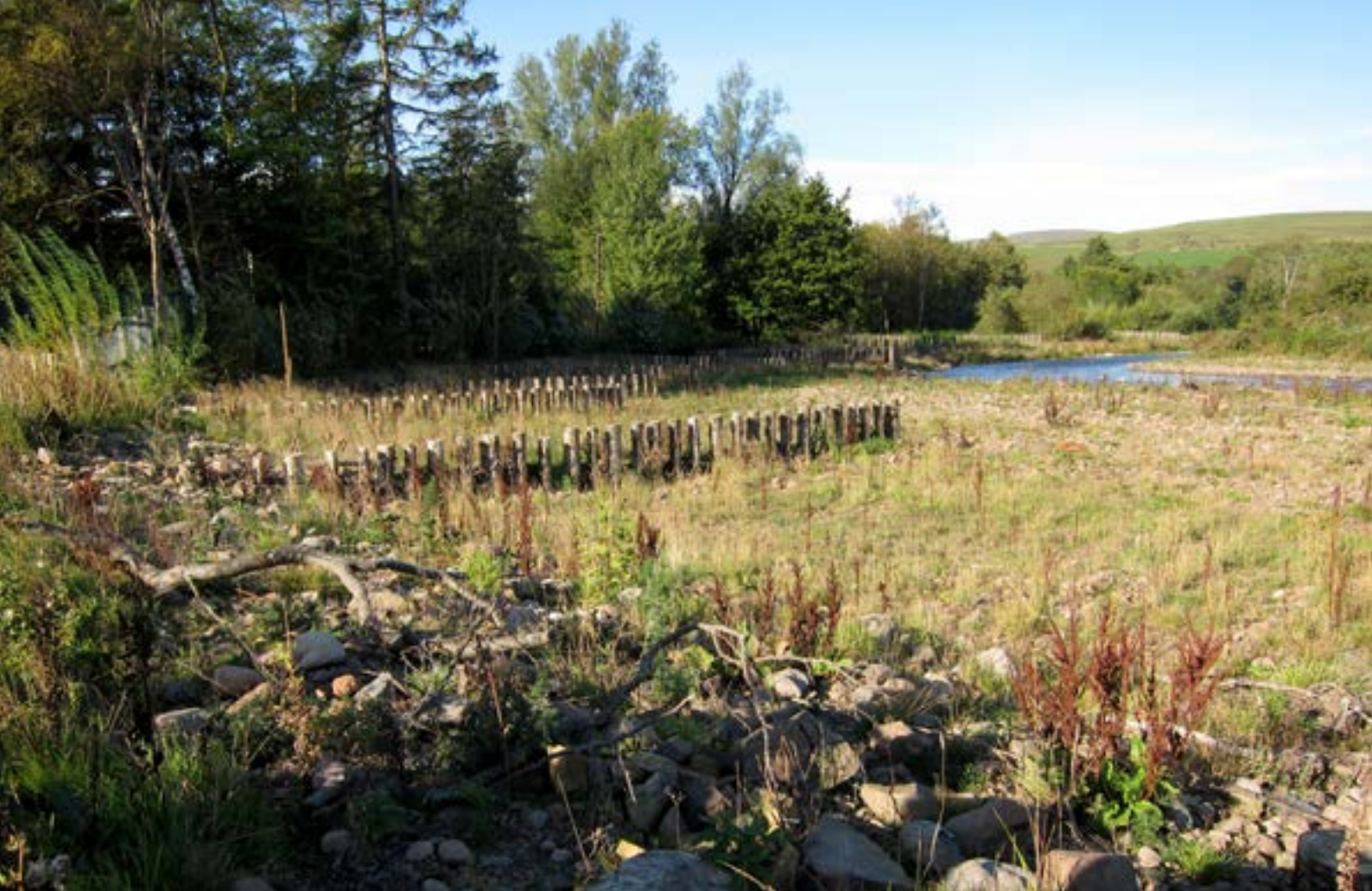
'Natural' timber posts to slow down water as part of flood management in The Cheviots. © Sarah Taylor
