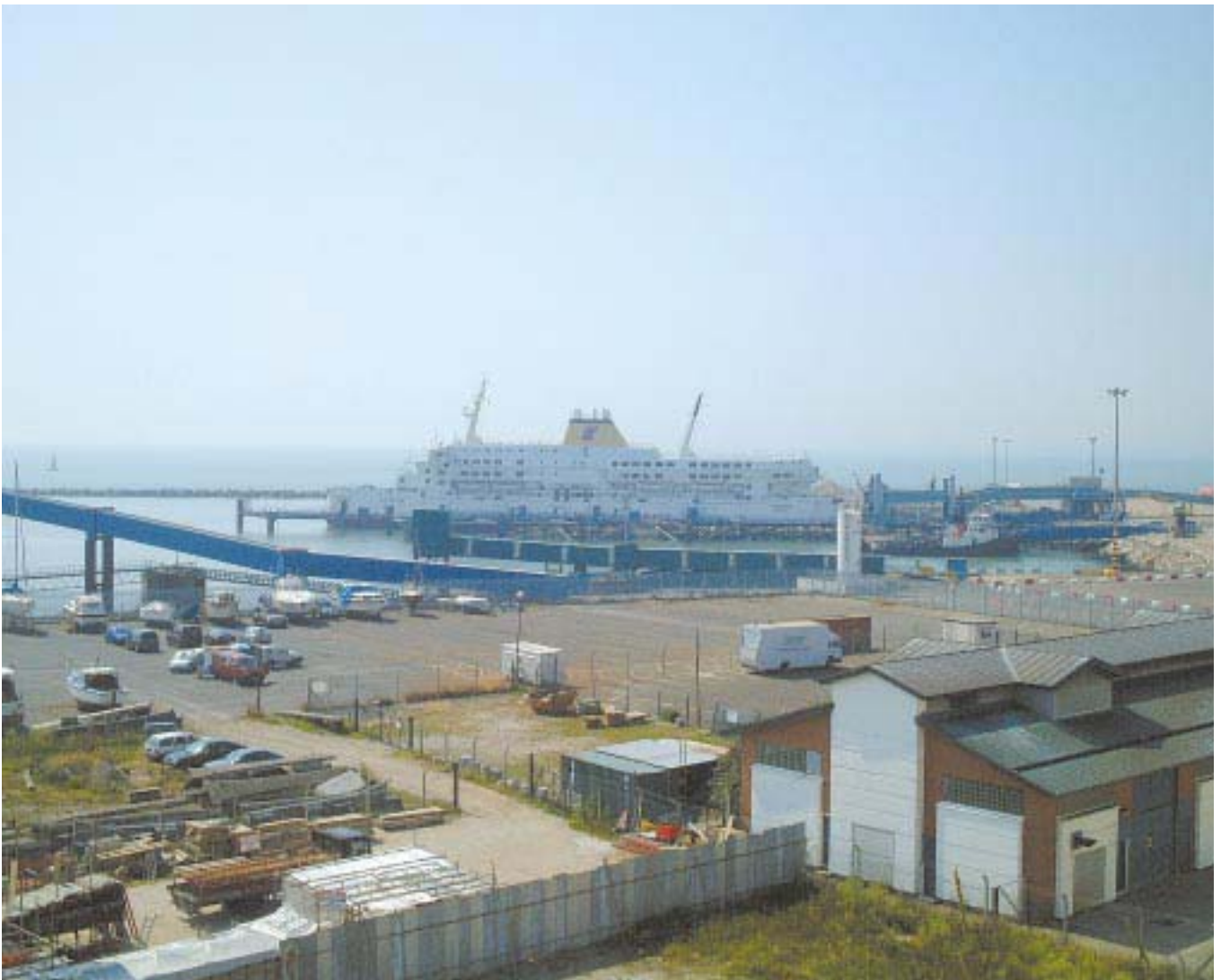
Major infrastructural developments are often located by the sea, such as Ramsgate port. Dan Laffoley/English Nature
