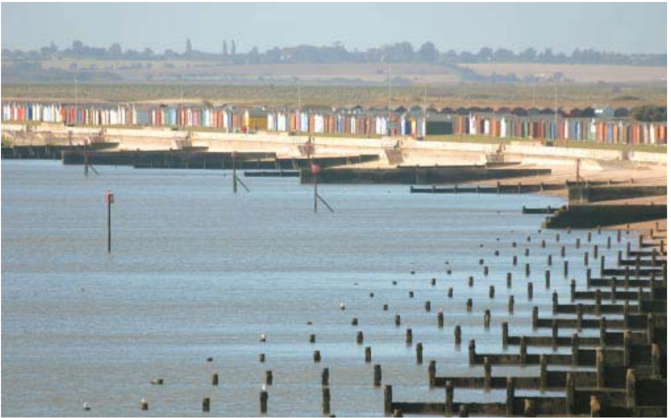
Groynes such as these at Dovercourt Bay in Essex interrupt the coastal processes and can lead to some areas being starved of sediment. Chris Gibson/English Nature
