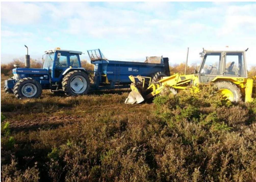
Loading of donor heathland plant material for transport to the restoration site
