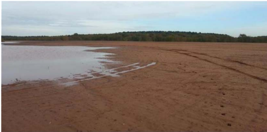
Newly placed sand substrate over colliery spoil
