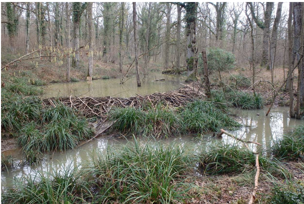
Figure 4. An impressive dam of approx. 20m in length in woodland in the Frome sub-catchment (territory 'Frome 6'). © A. Rothwell
