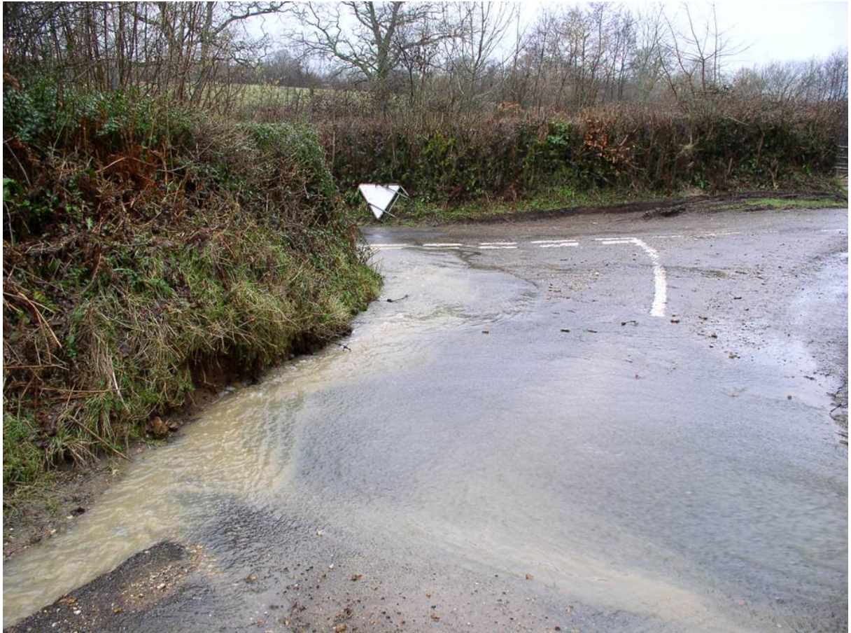
Figure 12: Photo showing damaged road verges and roads acting as a sediment pollution pathway in the Axe catchment (source J. Hickey, 2012).
