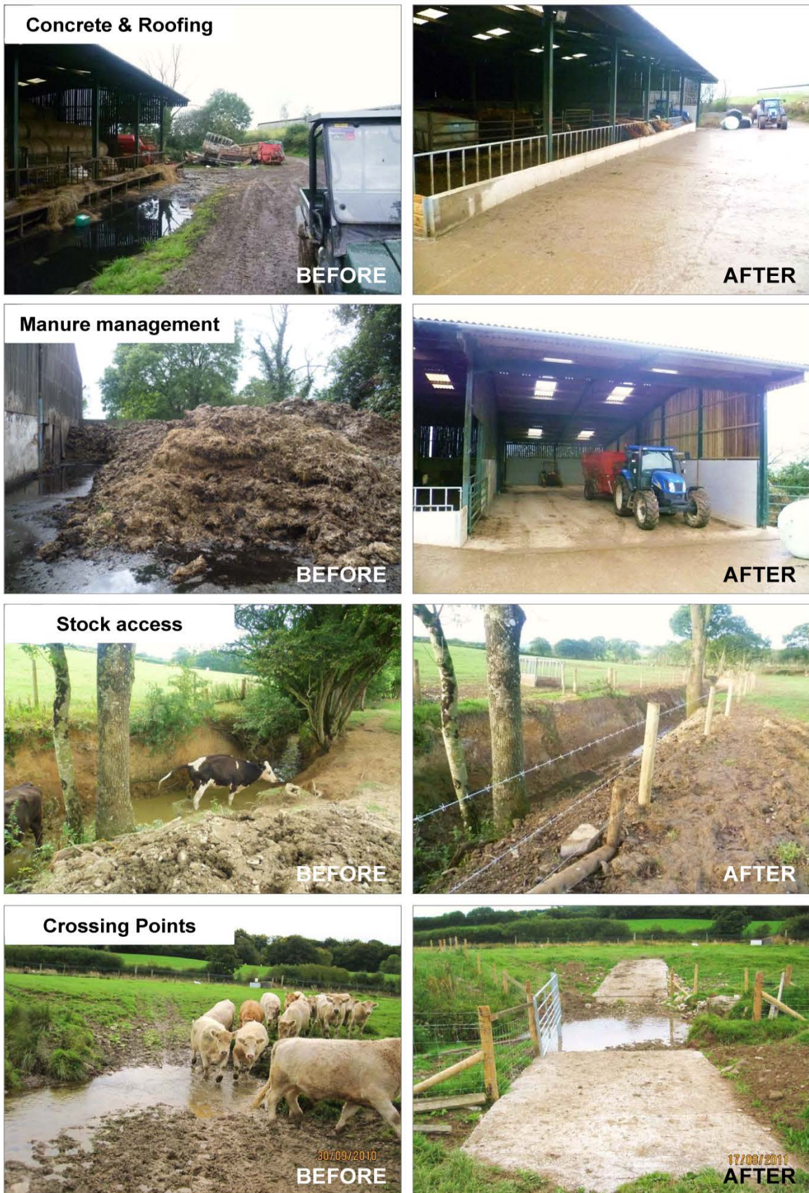
Figure 38: Actual examples of Best Farming Practices (BFPs) that can minimise loss of pollutants to watercourses as a result of agricultural activity.
