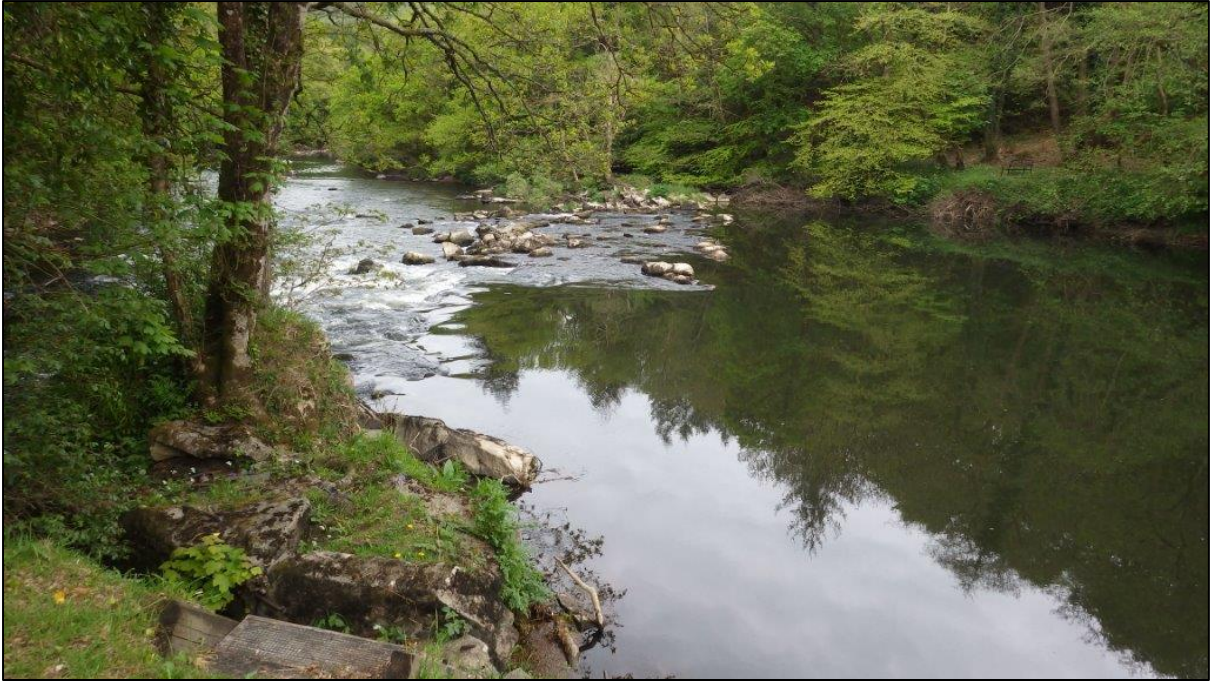
Figure A39. SX4197172519. Boulder weir across channel. Viewed from Devon bank, looking downstream.
