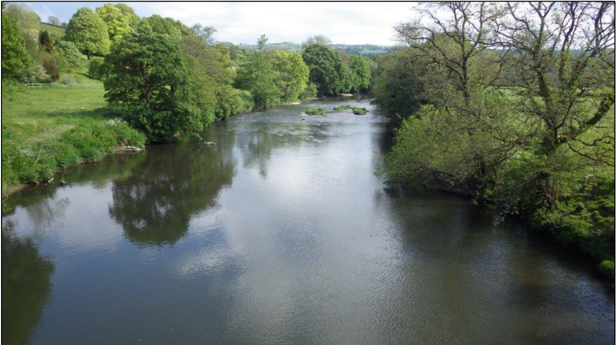
Figure A86. SX4000874872. View downstream from Horsebridge road bridge.
