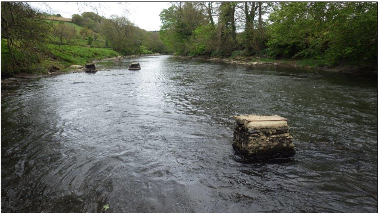
Figure A52. SX4064273985. Numerous fishing croy standings in channel along the Devon bank. Viewed from channel looking downstream.
