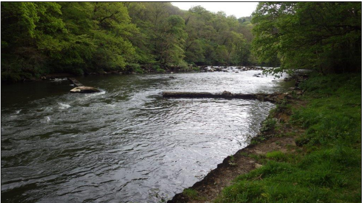
Figure A38. SX4205972515. Foreground: Double fishing croys. Background: boulder weir across entire channel width. Viewed from Devon bank looking upstream.
