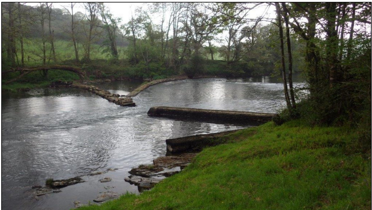
Figure A46. SX4148273332. First weir immediately upstream of Duchess Weir, adjacent to Weir Cottage. Barrier probably passable to shad due to laminar flow over shallow weir face. Viewed from Devon bank looking upstream.
