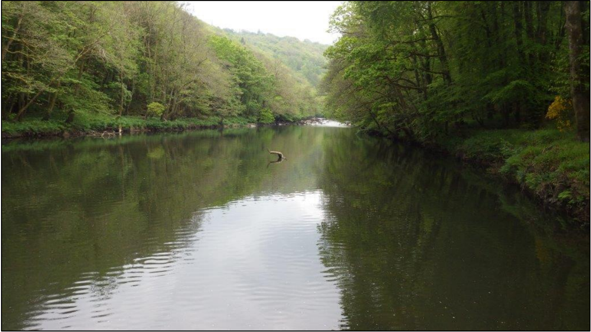
Figure A31. SX4263472515. Impounded water at Blanchdown EA Gauging Station. Viewed from channel looking upstream.
