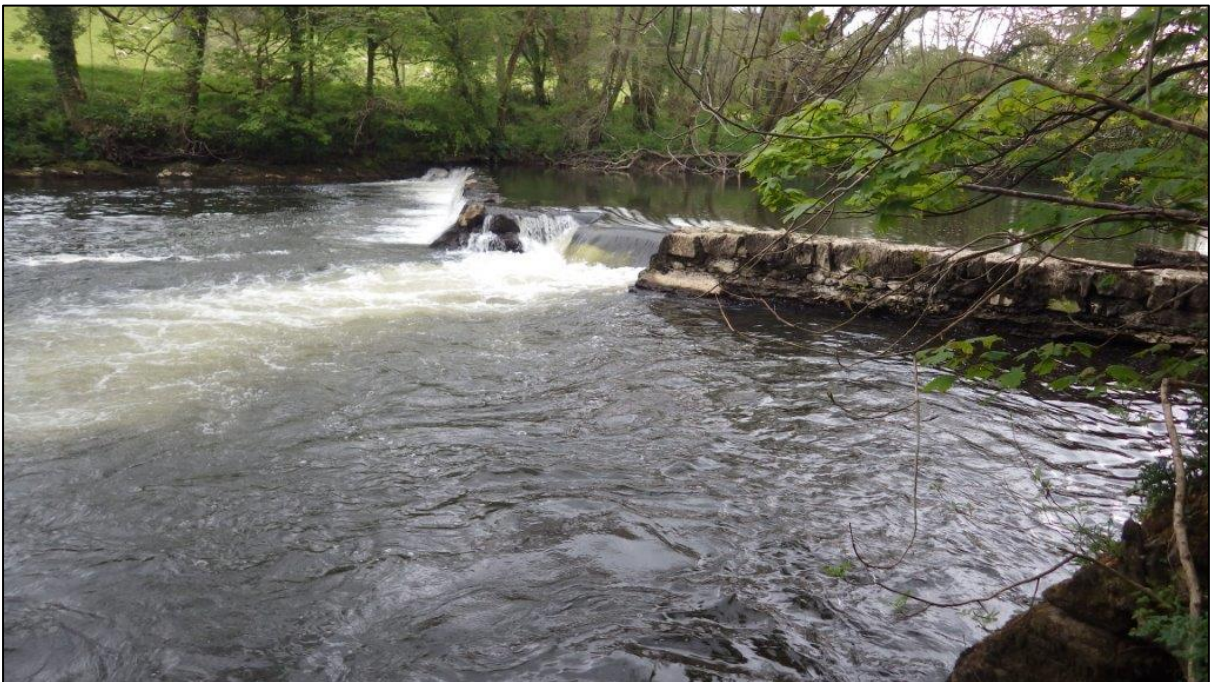
Figure A44. SX4150273203. Duchess Weir. Significant migratory barrier to shad. Viewed from Devon bank.
