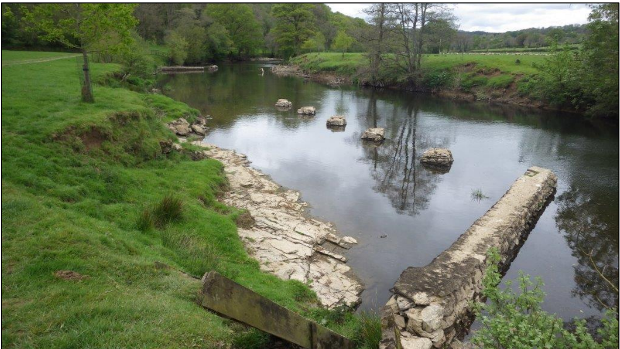
Figure A80. SX4000874118. Fishing croy and bedrock on Devon bank and platforms in channel. Viewed from Devon bank looking downstream.
