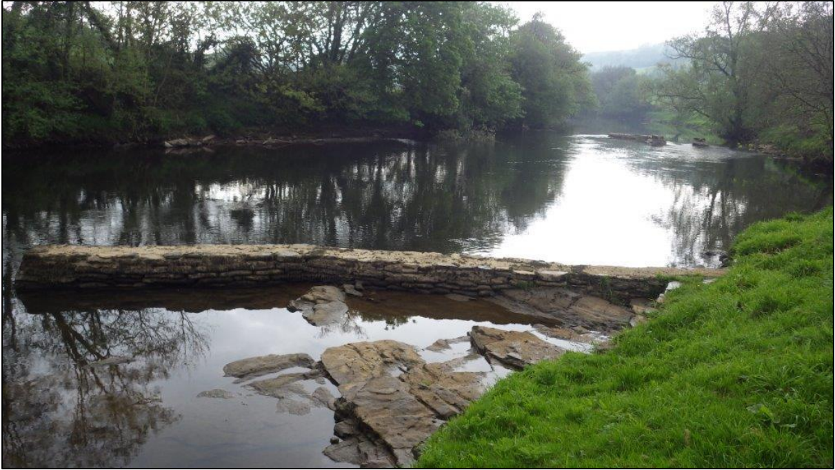
Figure A51. SX4134073777. Single arm, large fishing croys in the channel, background and foreground. Viewed from Devon bank looking upstream.
