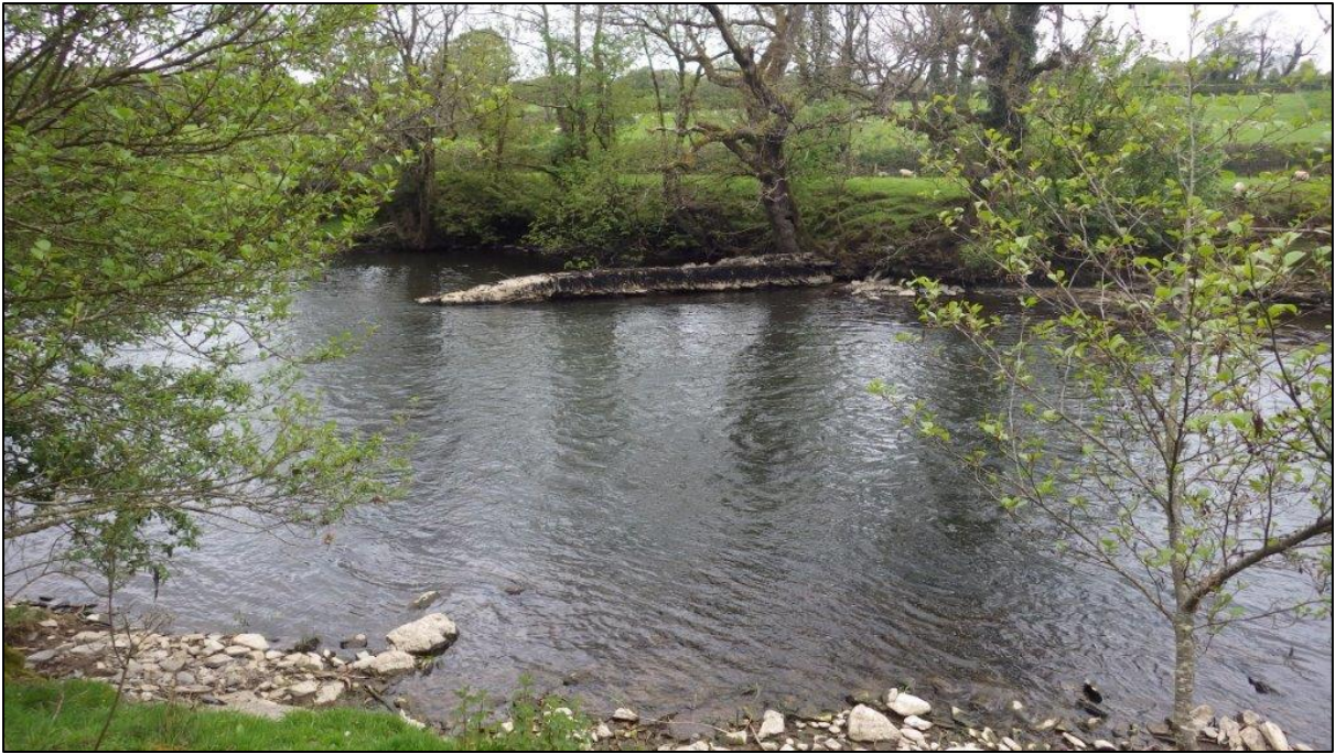
Figure A75. SX3958673923. Fishing croy on Cornwall bank downstream of Lamerhooe Weir.
