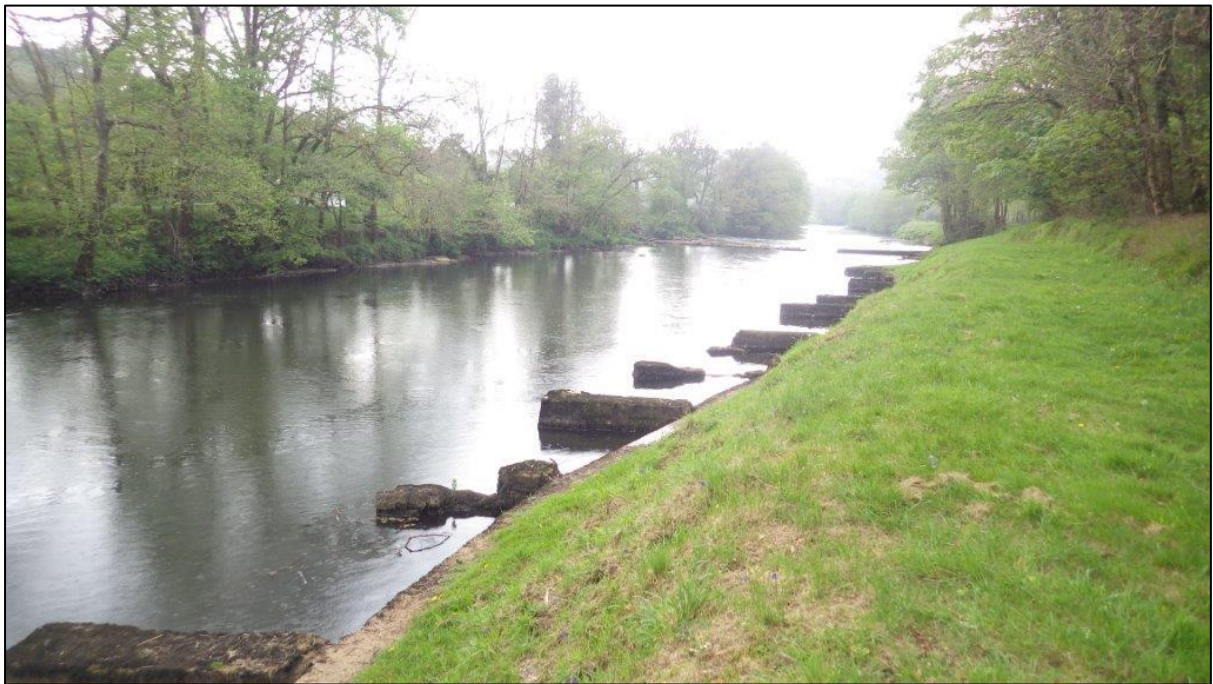
Figure A45. SX4150173212. View upstream from Duchess Weir. Fishing croys along Devon bank and another weir in the background.
