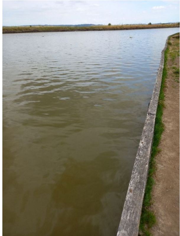
Photo 9. Large Moat - E1. © Abrehart Ecology 2023
