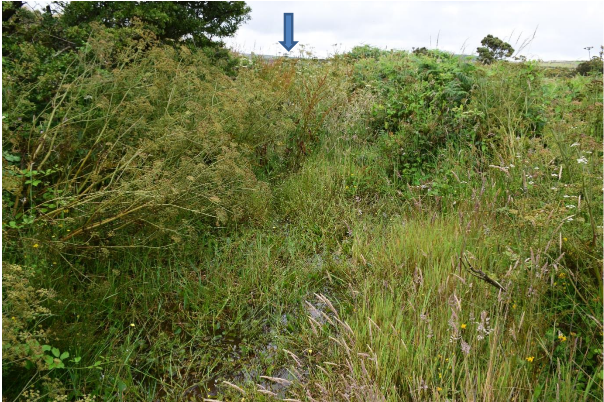
Photo 9. The end of the track leading to the gate (arrowed). The rank vegetation around the gateway suggests it is no longer in use.
