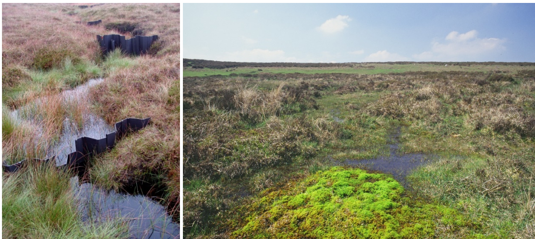
Picture 4.2 Grip blocking techniques use to raise water levels. Plastic has been used to block the drains or grips, but now natural materials, such as bales, brash, wood and peat is preferred. Left photo © Natural England/David Glaves; right photo © Natural England/Peter Wakley
