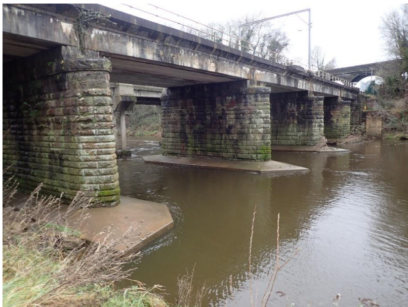
Figure 11: The bridge supports of the railway line at NX 38861 57058
