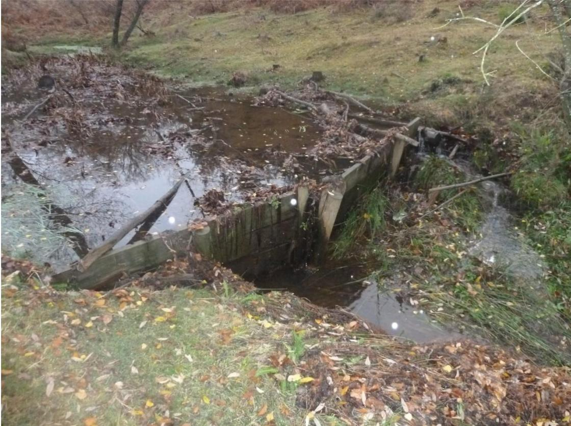
Figure 1-10: Wooden weir structure
