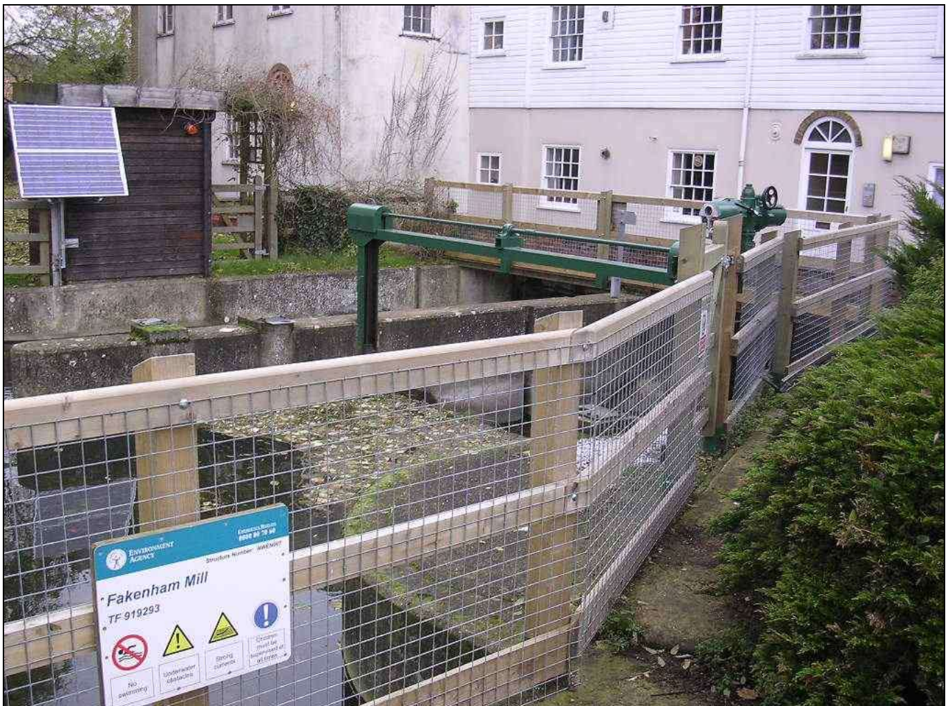
Plate Bk1 View upstream of weir at Fakenham Mill
