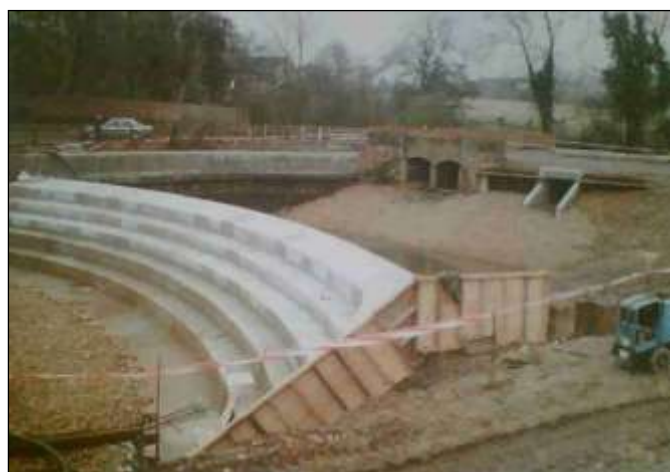
Plate Bb1 Left: Automatic tilting gate within Costessey Mill: Right: Costessey horseshoe weir under construction
