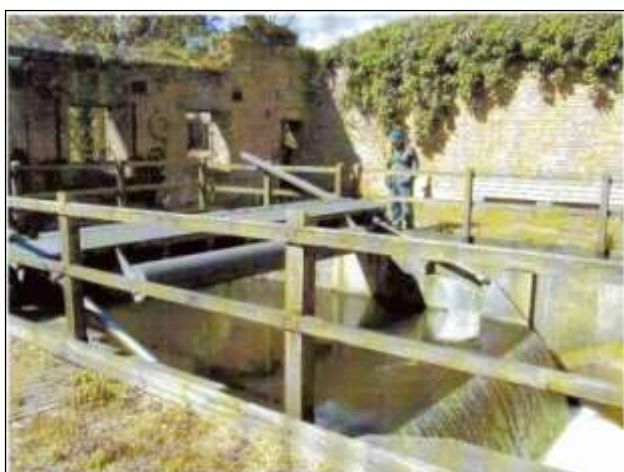
Plate Bb1 Left: Automatic tilting gate within Costessey Mill: Right: Costessey horseshoe weir under construction
