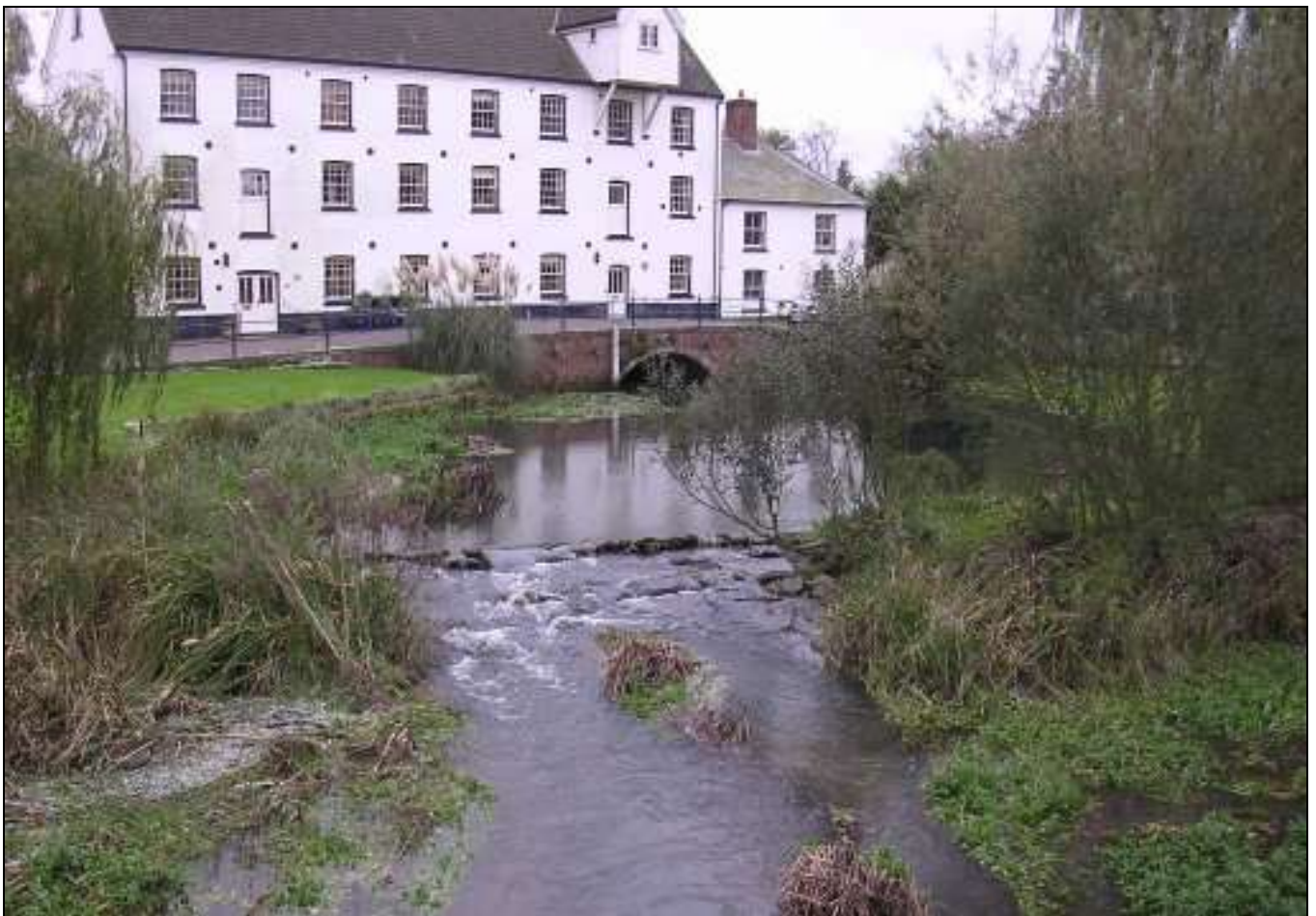
Plate Bd1 View of Lenwade Mill from main road (downstream)
