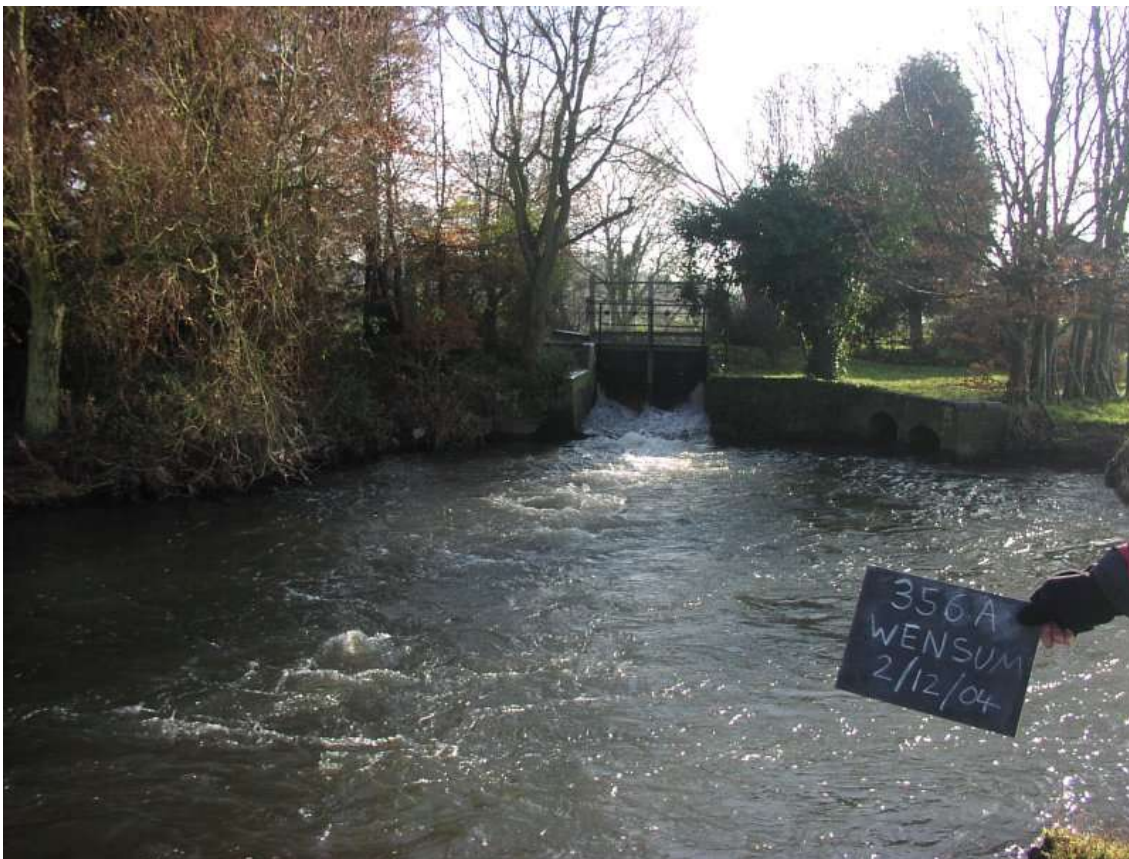
Plate Bf1 View of by-pass sluices at Elsing Mill from downstream (photo from GeoData, 2006)
