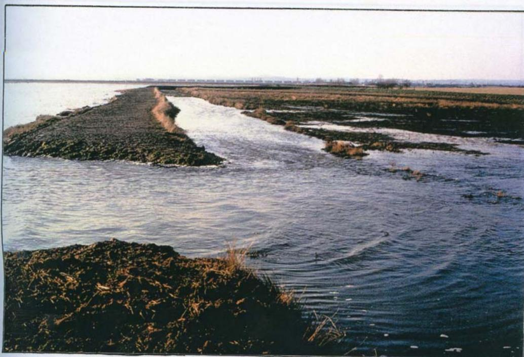
Plate 6. Early rising tide showing current flow around the edges of the spillway and into the front borrow pit
