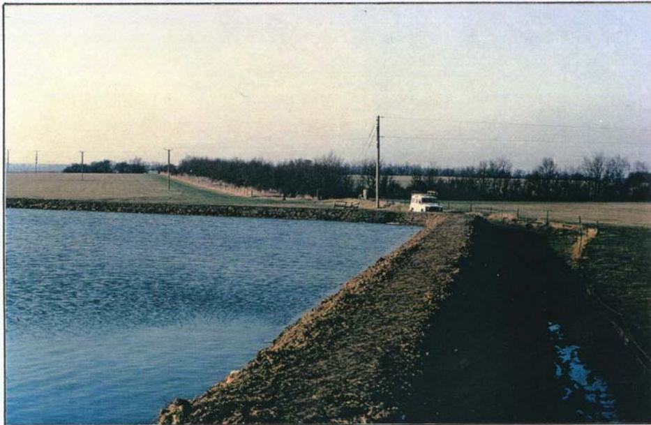
Plate 12. High tide at the east end of the site showing seepage through the eastern wall
