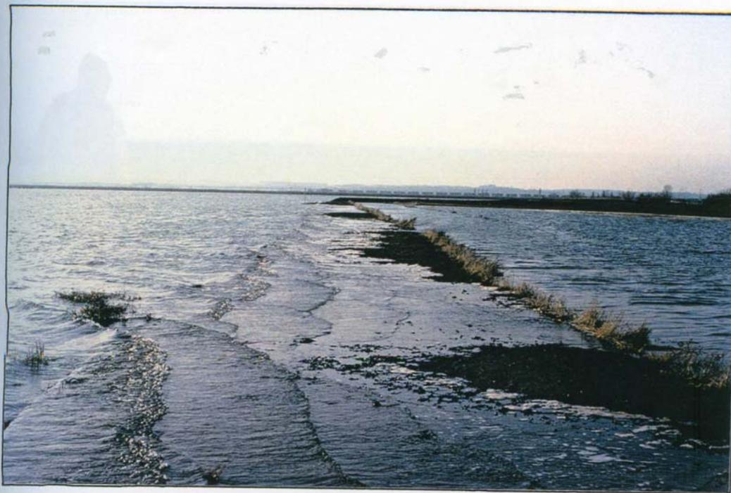
Plate 5. The surface of the set-back area is covered before waves break over the front wall
