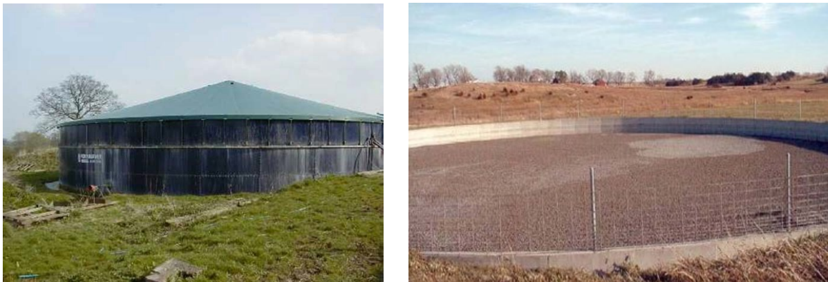
Figure 6. Slurry store covers; rigid cover on above ground slurry tank (left) and floating cover of expanded clay granules (right)
