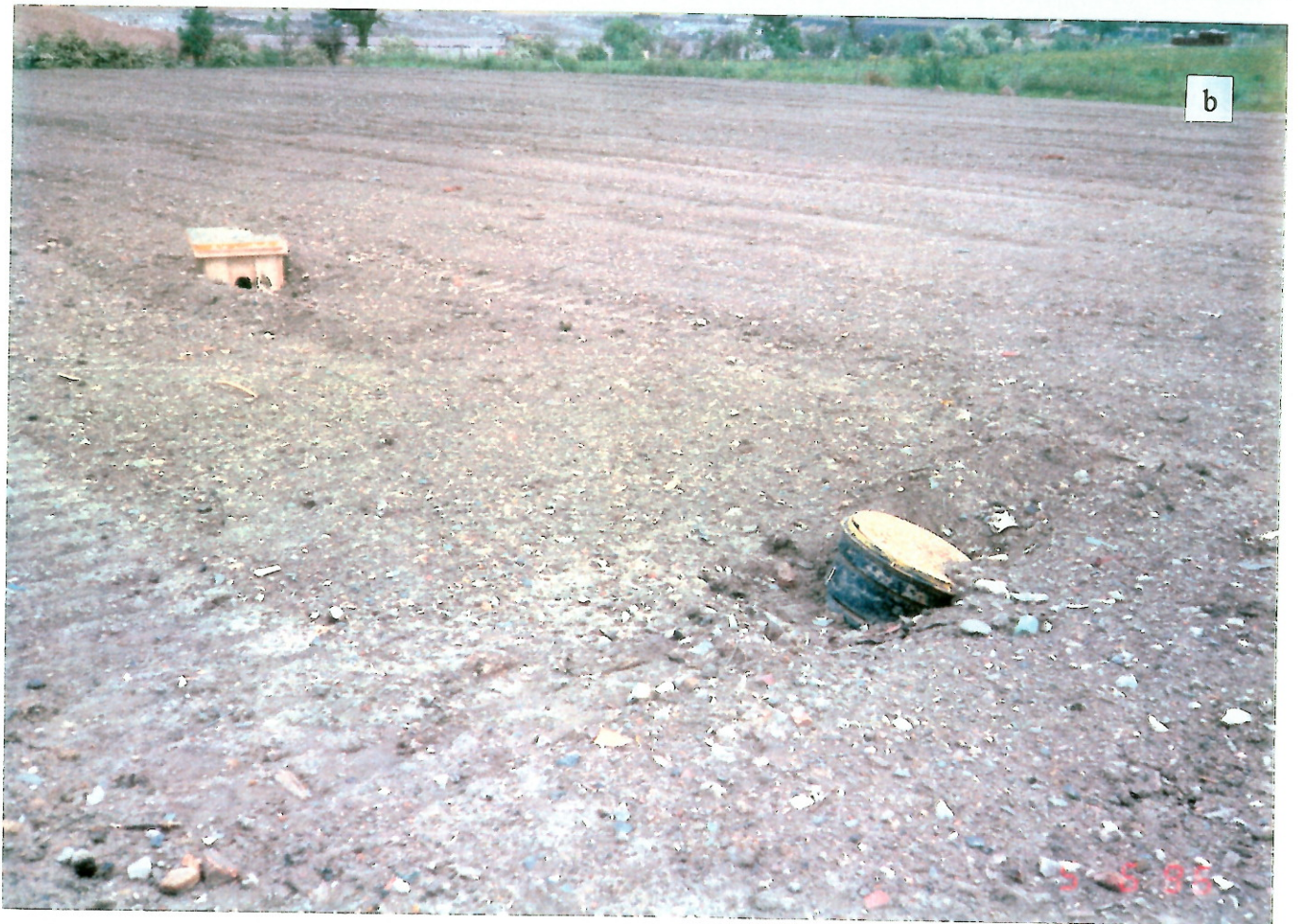
The area of subsidence recently re-engineered and raised with imported material.
