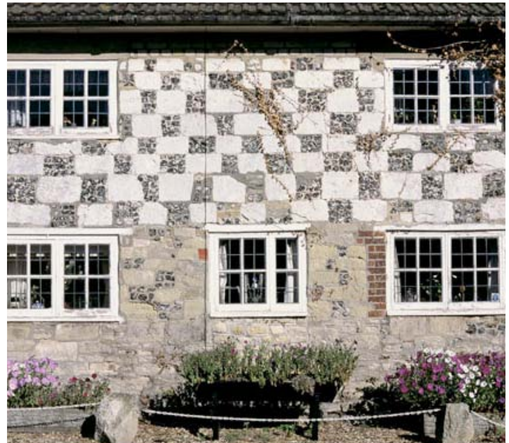
Typical house front in the Wylde Valley.
