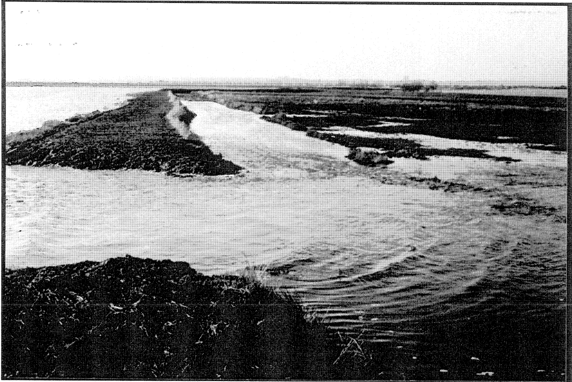
Plate 9: January 1992 View across the spillway showing wave diffraction patterns and current flows into the front borrow pit before this was filled
