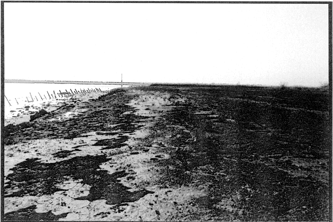
Plate 14: February 1994 Looking along the front wall from east to west showing flaking of surface sediment layers
