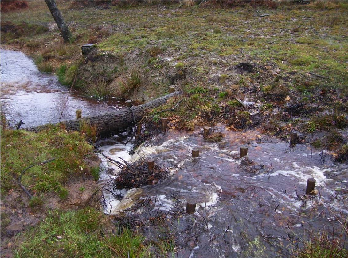
**Figure 1-4: Existing restoration measures to combat erosion: low weir, posts and heather bales on the outflow channel from Buckherd Bottom (NGR 420717 108488)**
