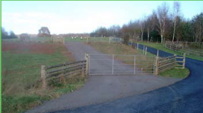
Access track and gateway after CSF grant work
