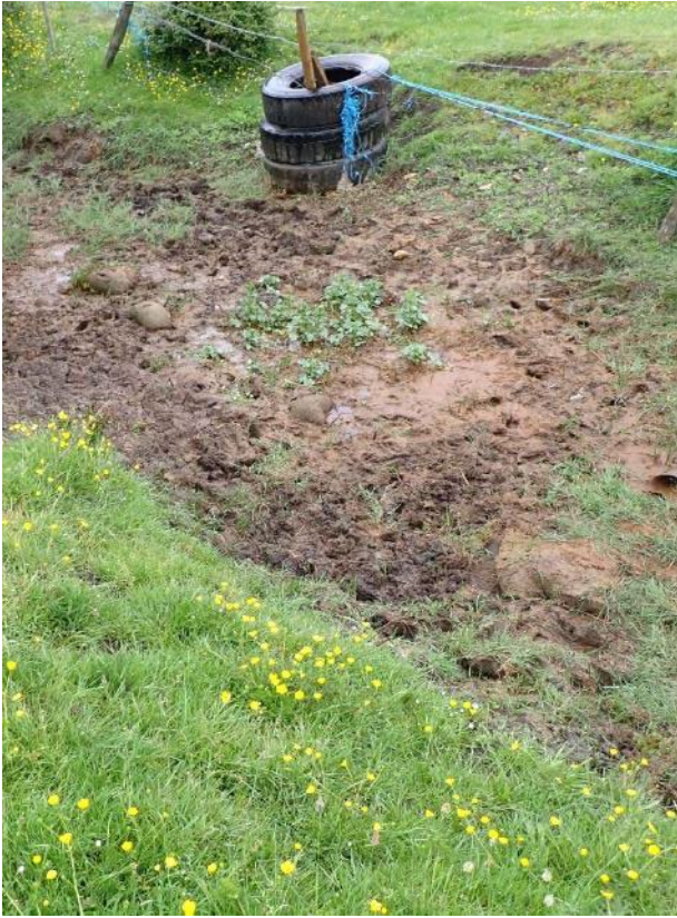
Photo 17. Drying ditch – TFM6.
