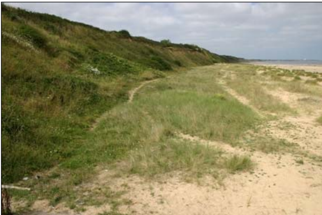
Photograph 7 Sandy grassland at the limit of the sea wall stretching below the low cliffs and towards Lowestoft. The beach reduces the impact of wave impact on the cliff face and it has become vegetated.
