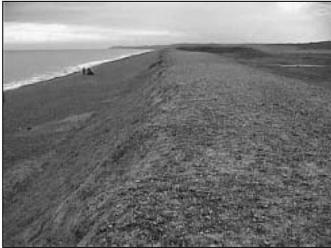
**Figure 03-01a** An artificially reprofiled beach at Cley North Norfolk, October 2001. The picture was taken looking southeast along the coast.
