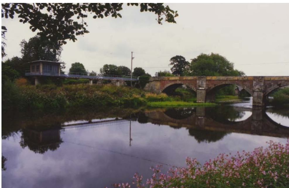
Plate 3.2 Gauging station, River Vyrnwy at Llanymynech. The instrument building, housing a water level logger, can be reached by a catwalk at times of overbank flow. The station is calibrated using a current meter suspended from a cableway.
