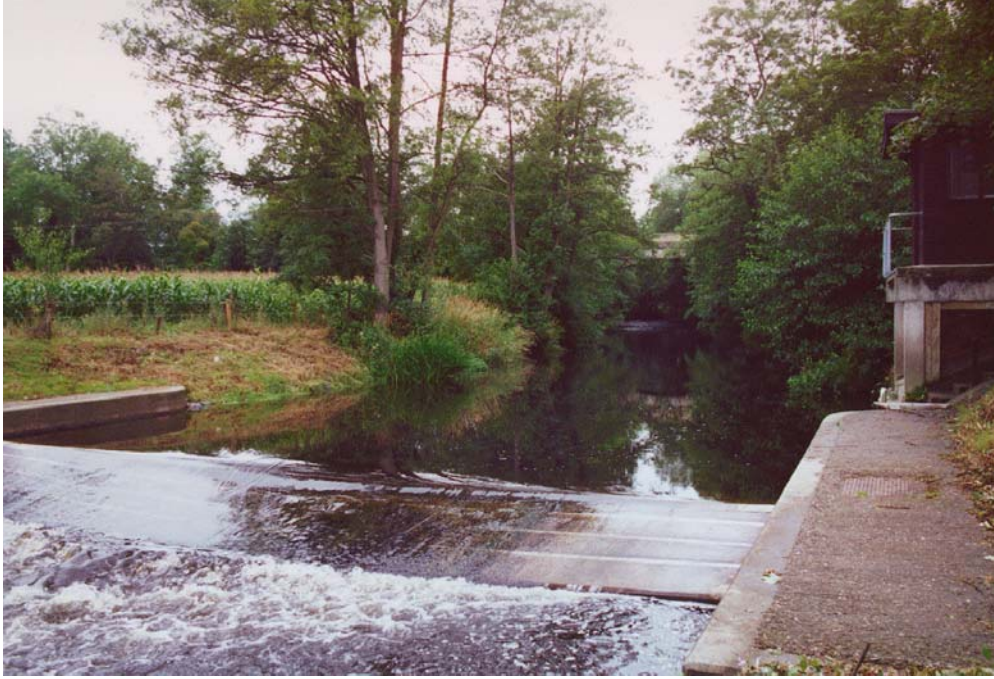
Plate 3.3 Gauging station at Llanfyllin, a flat-V weir with a precise rating of discharge versus depth
