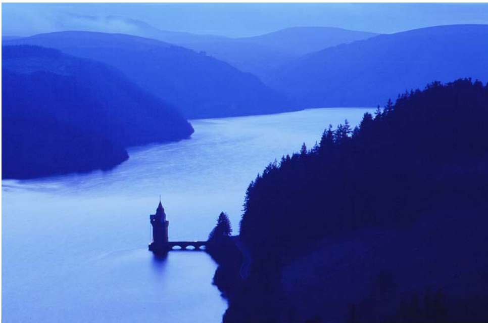
Plate 2.1 Lake Vyrnwy, constructed as a water supply reservoir for Liverpool in the 1880s, has an area of 4.45 km 2 and now also has a role in regulating the flow of the Severn (Photo courtesy of Altered Light).
