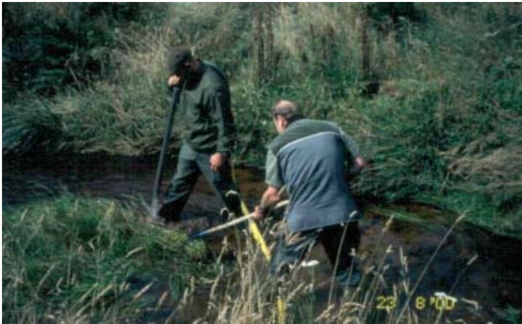
Cleaning gravels to enhance the riverbed for salmon – undertaken by the EA
