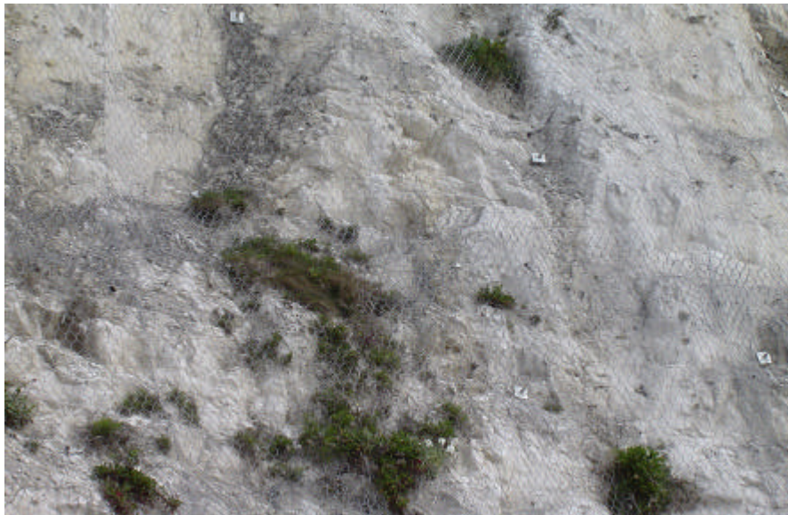
Figure 5. Detail of recent ‘mesh’ on the chalk at Black Rock. It shows early stages of vegetation growth and accumulation of debris behind the ‘mesh’. Natalie Bennett/ English Nature.
