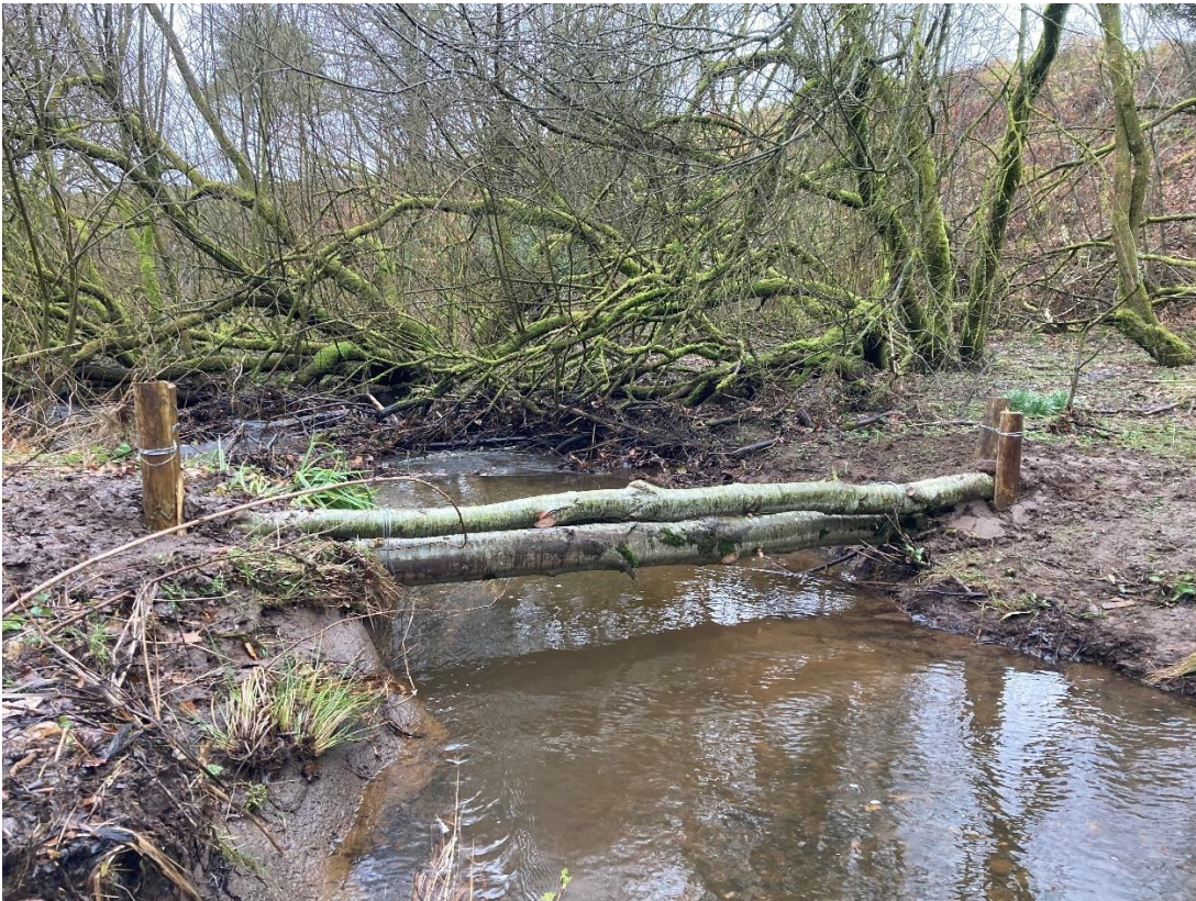
Wye leaky dam at Derwent Living Forest. Photo credit Daniel Blake.
