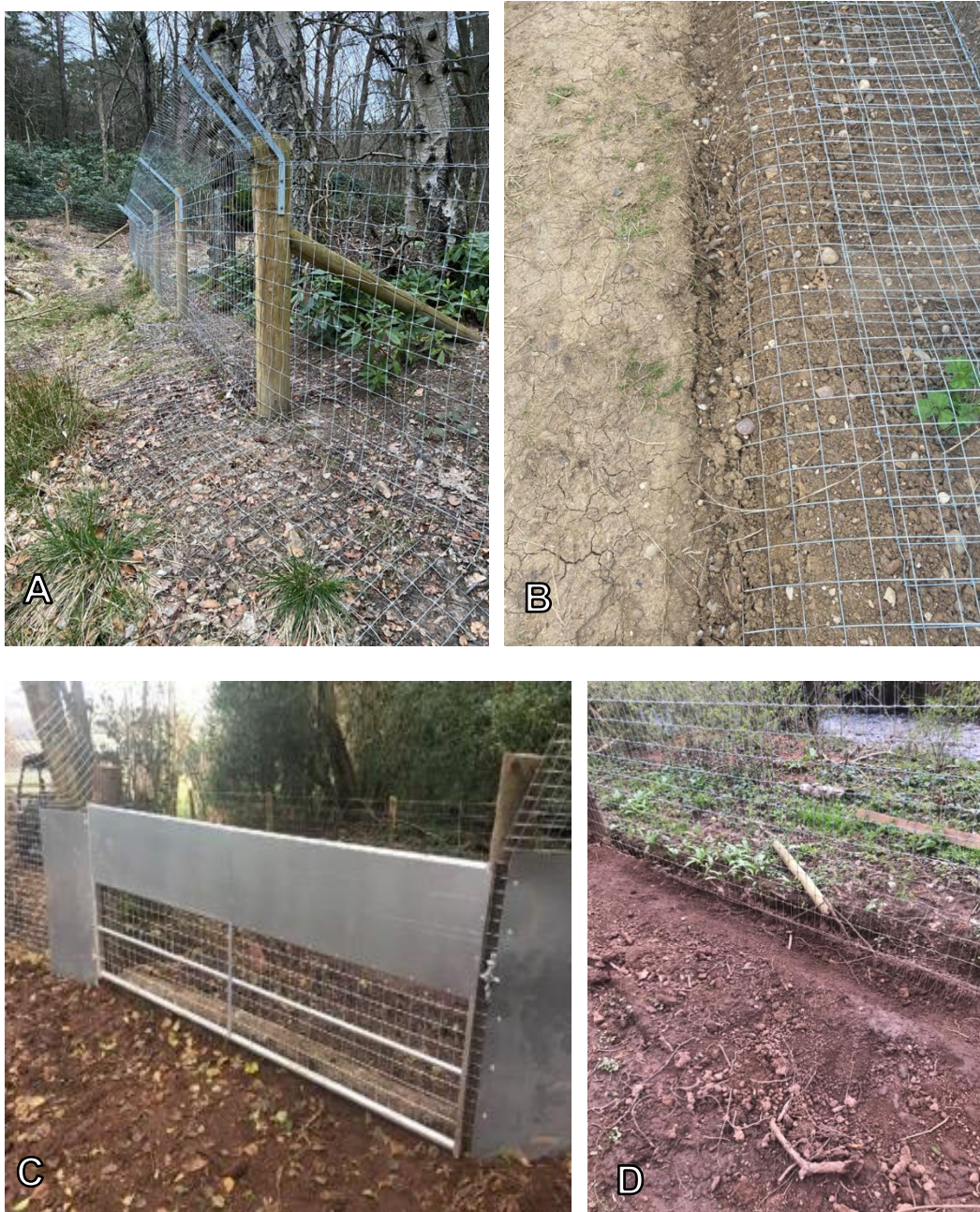
Figure 15: A: Beaver fencing showing an overhang and 90cm mesh skirt; B: an example of fencing with mesh skirt which is also then buried beneath the ground; C: an access gate with overhang and anti-climbing metal where overhang not possible, noting gate is also set on a concrete plinth to prevent digging; D: showing repeated fence pacing and digging behaviours which should be regularly monitored and appropriate management action taken (highly motivated by close proximity of fencing to an external water course). Photo © R Campbell-Palmer, Beaver Trust.
